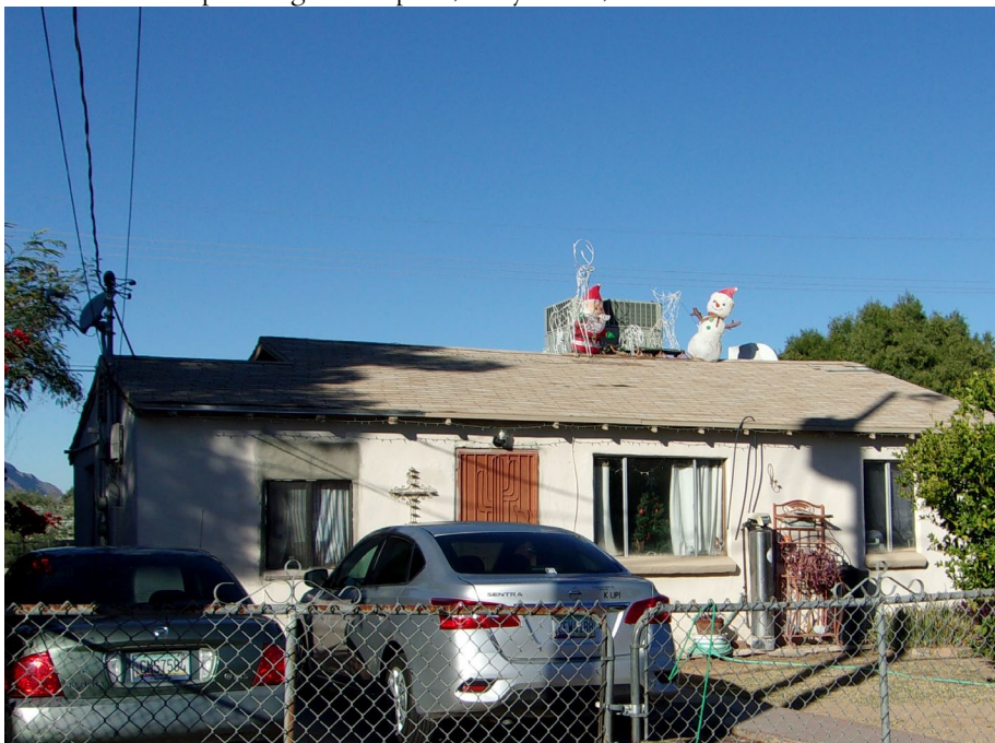
Exterior of Ms. Glenn's lead safe property and her new roof.
