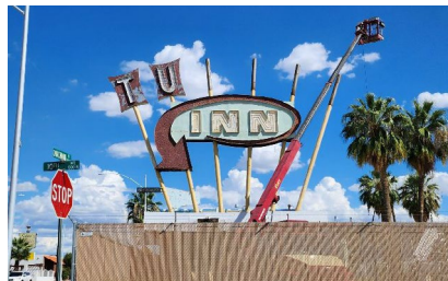
Tucson Inn sign before and during construction.
