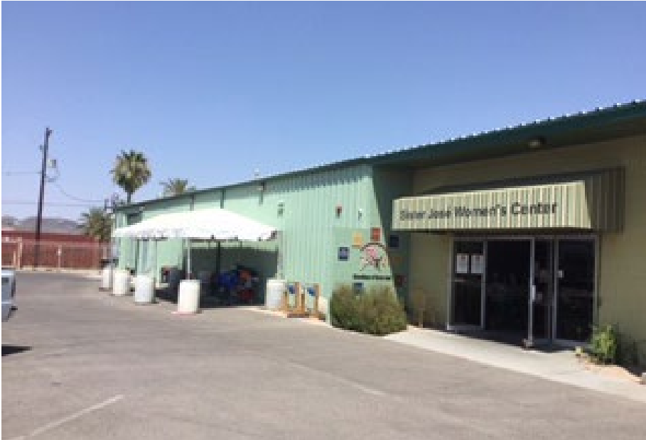
Before exterior of Sister Jose Women's center before installation of solar panels.
