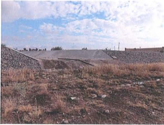
Outfall 101-16.74 - Looking southeast towards east bank of New River
