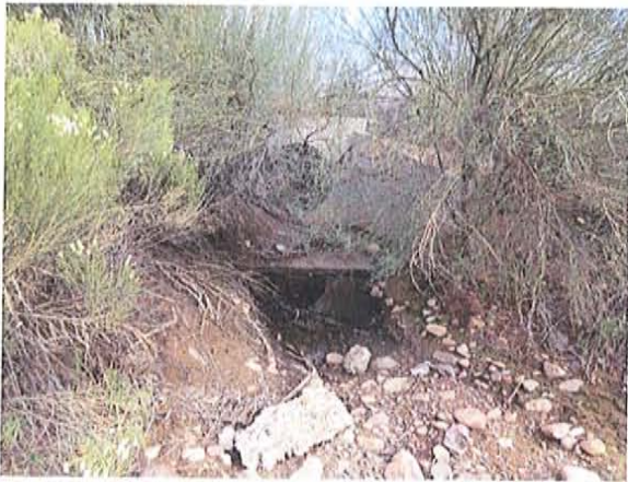
Outfall 101-16.31 - Looking east into east bank of New River
