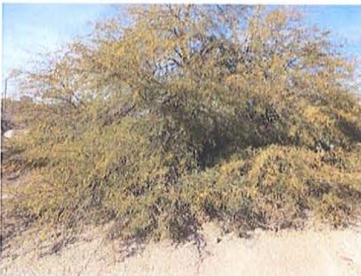
Tree covering outfall
