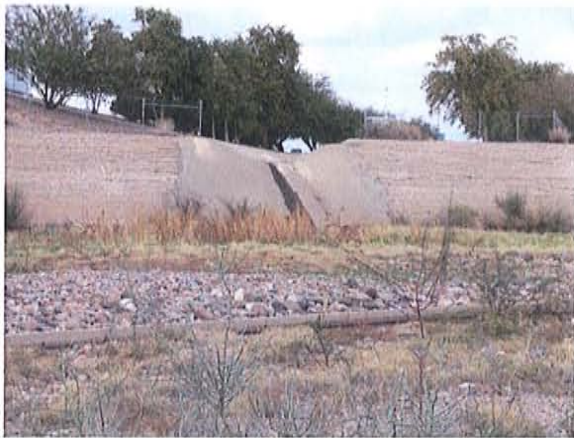
Outfall 101-13.68 - looking north at outfall on north bank of Skunk Creek
