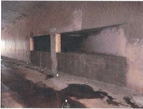
Outfall 202-3.57 - Looking northeast into outfall under 202
