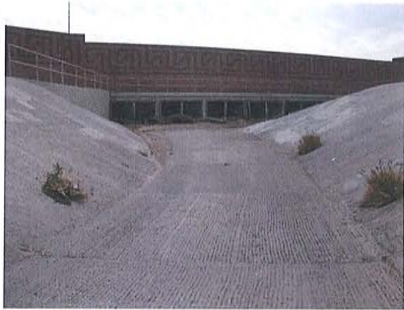
Looking southwest at outfall 60-189.65
