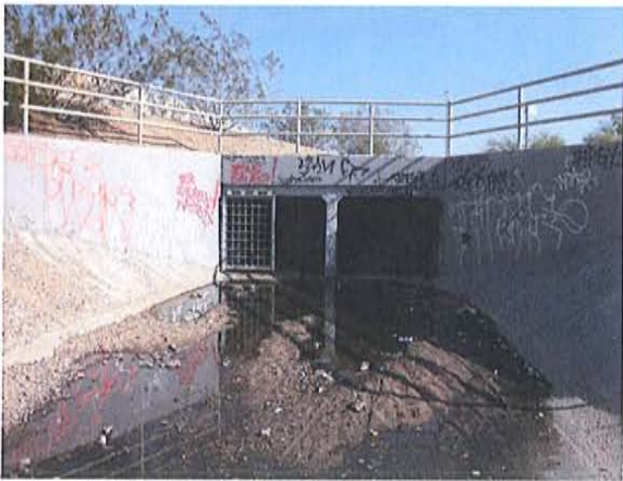
Outfall 101-25.92 - Looking east into the outfall
