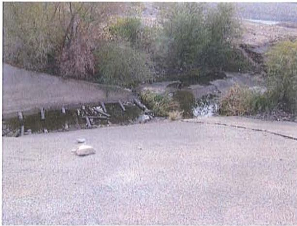
Looking southeast at outfall 10-149.18
