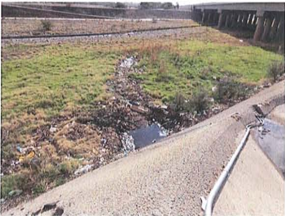
Debris at base of outfall (looking south from outfall)
