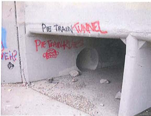
Outfall 101-21.23B - Looking at outfall on east side of underpass.
