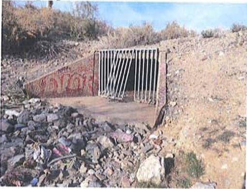
Outfall 51-8.22 - Looking north at outfall
