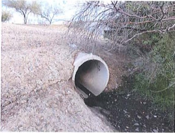
Outfall 101-20.19 - Looking North towards River Bank
