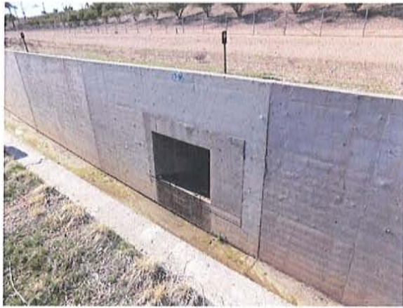
Outfall 143-2.90 - Looking southwest into canal
