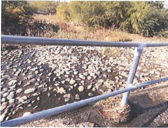
Looking north at outfall 101-10.84
