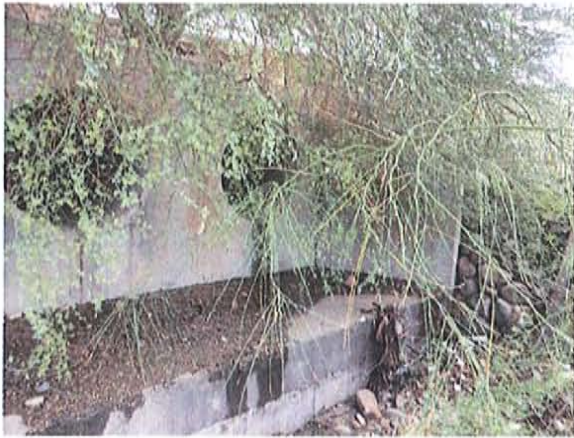
Looking south at outfall 101-13.44
