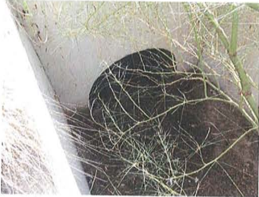
Outfall 10-150.06 – Looking southwest
