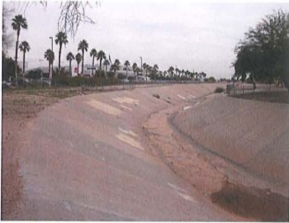
Looking east at outfall 60-187.43
