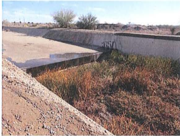
Looking southeast at outfall 101-7.76
