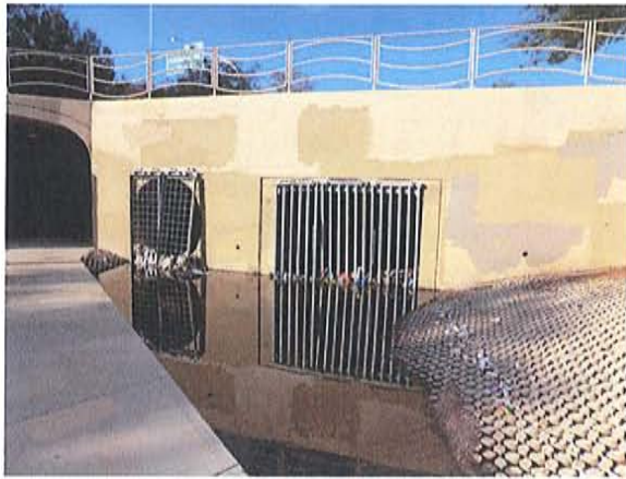
Looking northwest at outfall 51-11.62
