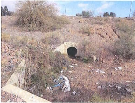
Looking east into outfall 101-15.18 east bank of New River
