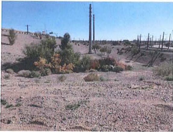
Outfall 202-5.14 - Looking south towards open channel
