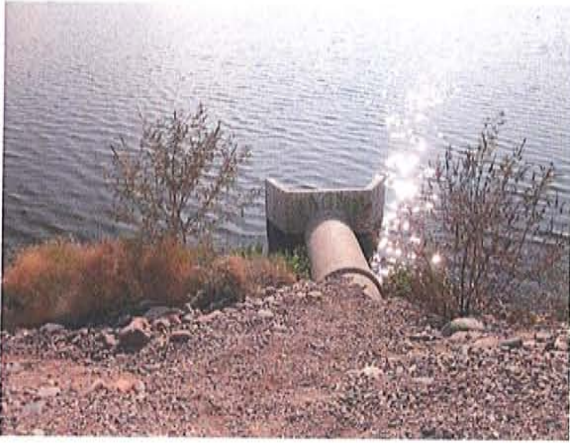
Outfall 202-8.65 - Looking south into Tempe Town Lake
