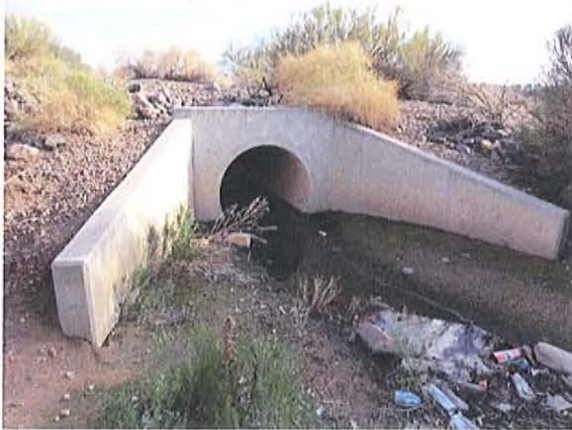
Outfall 101-16.62 - Looking east into east bank of New River
