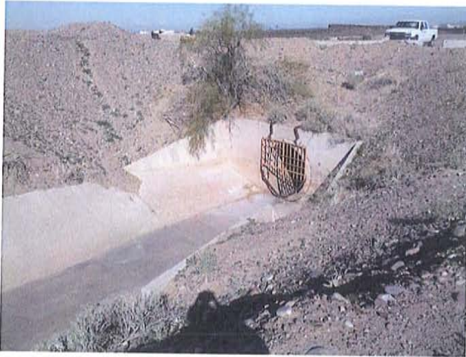
Outfall 17-198.48 - Looking north at the outfall
