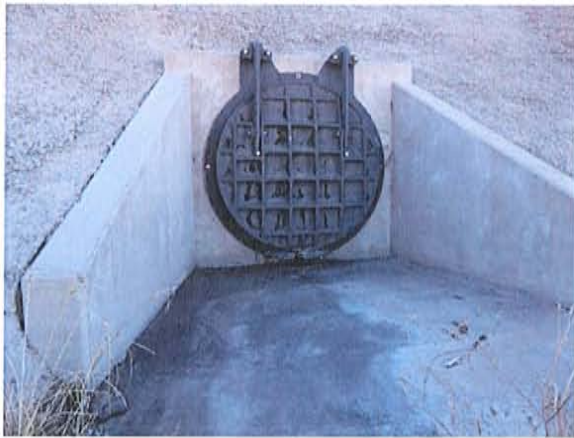
Outfall 153-1.64 - Looking south into outfall
