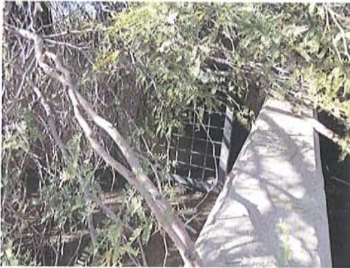
Outfall 51-7.04 - Looking north into the outfall
