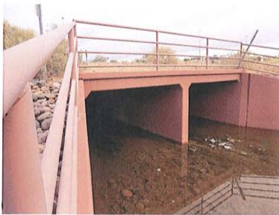
Looking southeast into outfall 10-162.44
