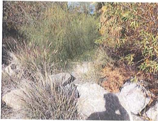
Heavy over growth around outfall
