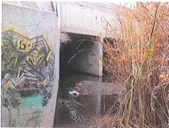
Outfall 101-51.07 - Looking southwest
