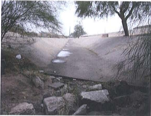
Outfall 101-21.87A - Looking east towards outfall
