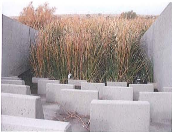
Outfall 202-14.22 - Looking north into outfall
