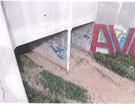
Outfall 101-50.87 - Looking northeast toward outfall
