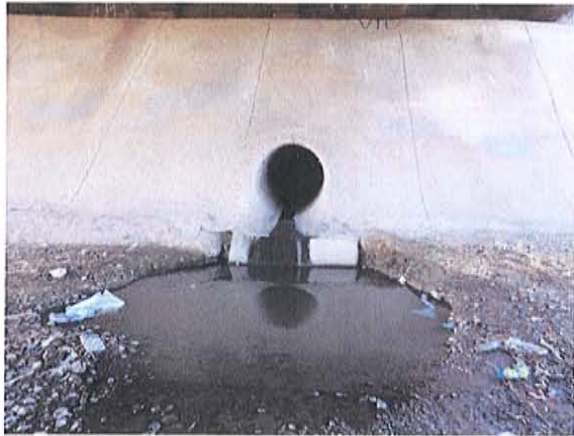
Looking west at outfall 10-130.20 under W. Van Buren
