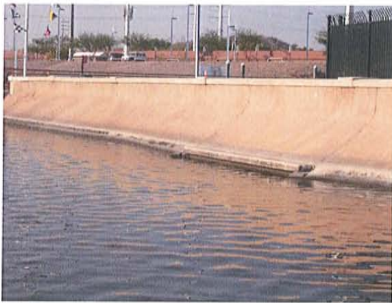
Outfall 202-7.44 - Looking to the northwest towards the north bank of Tempe Town Lake (outfall is underwater)
