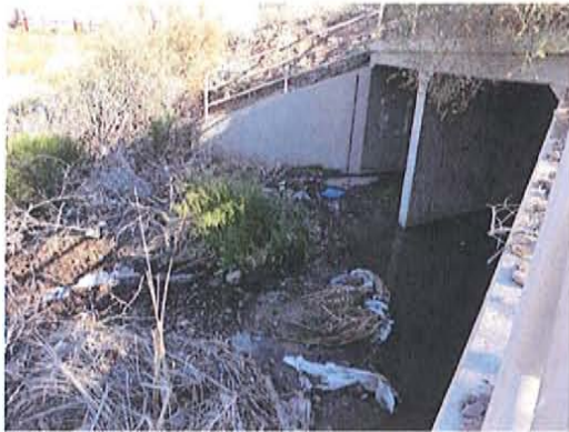
Outfall 101-11.85 with debris present
