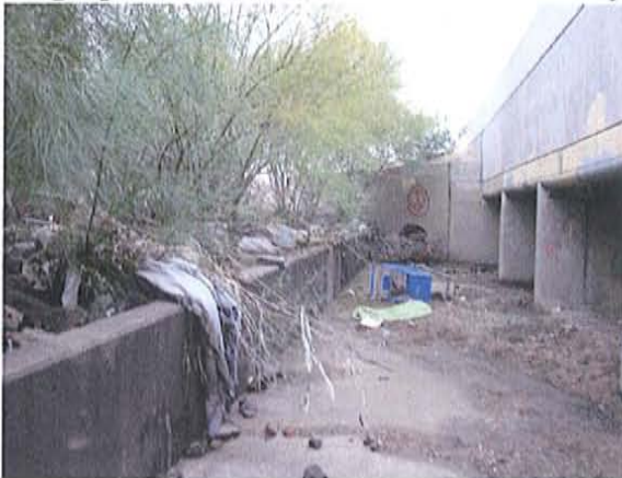
Outfall 101-21.87B - Looking east at outfall on east bank of Scatter Wash
