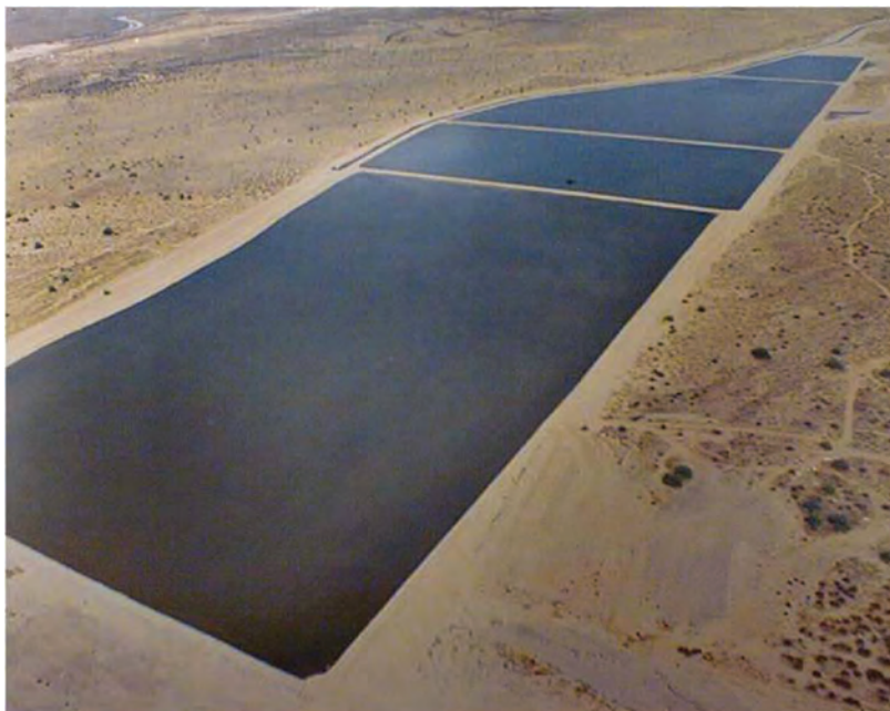
Spreading basins, such as the Granite Reef Underground Storage Project above, allow water to percolate into the soil and are used to recharge the groundwater tables.
